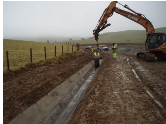
Concrete Canvas being applied to a channel: Courtesy of the Environment Agency
