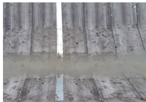
Figure 3. Stainless steel batten check slot
