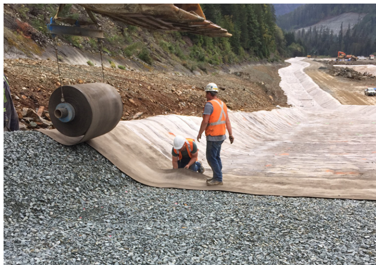
Figure 4. CC installed on a granular sub-drainage layer
