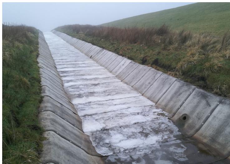
Figure 5. CC remediation with sub-drainage perforated pipe discharging at 10m centres along structure
