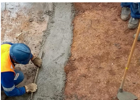
Figure 2. Poured concrete check slot being installed in channel
