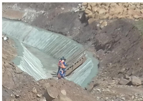
Figure 1. Section of channel at risk of boulder impact and potential damage
